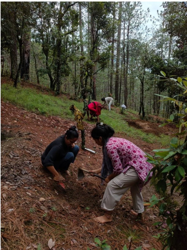
Trenching work underway on the slopes.
